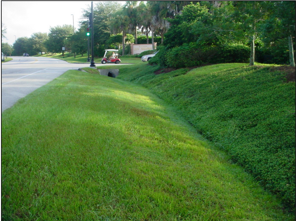
Drainage swale and pipe at Rio Grande Avenue
